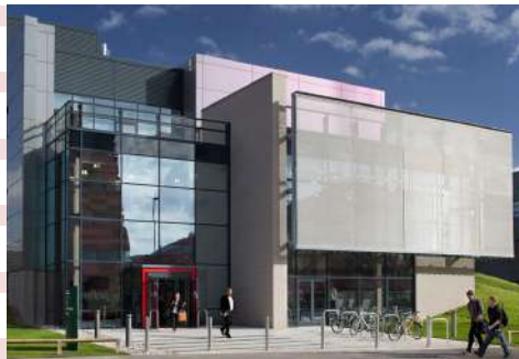
BREEAM Outstanding Energy Technologies Building Nottingham
