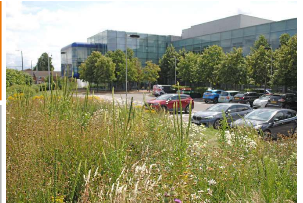
BREEAM Very Good Swindon & Wiltshire Building Swindon
